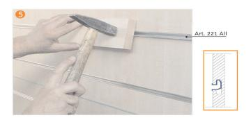
5º When the lower panels have been put in place, insert the horizontal profiles by using a rubber mallet or a hammer with a buffer.
